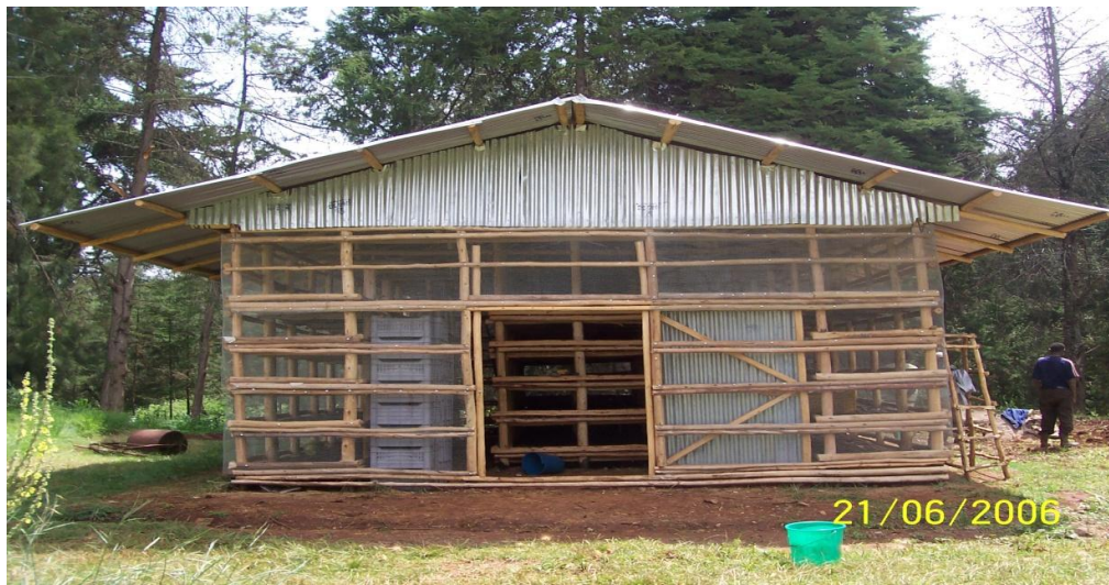
Fig. 2. Diffused light store constructed at Holetta research center
